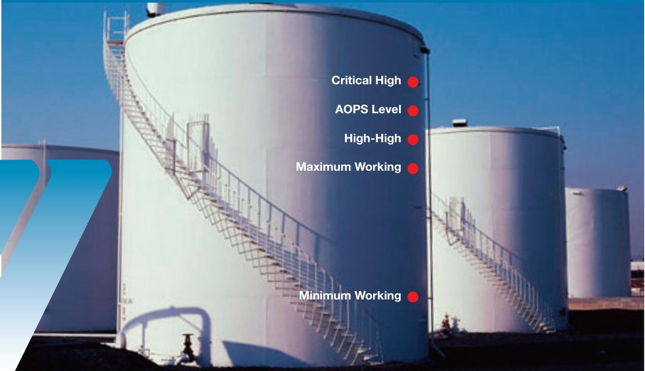
Levels of Concern are calculated product levels in the tank upon which all alarm and alert positions and response times are based. Careful calculation of LOCs ensures the success of the OPS.
